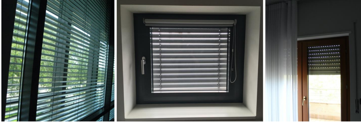
Figure 3: Different examples of window shades/blinds: Automated perforated Venetian blinds in office with automated control (and manual override)(left); Residential blinds with manual control (center); Internal curtain and external roller shades in dwelling.
