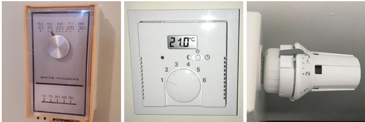
Figure 4: Examples of residential building thermostat interfaces.
