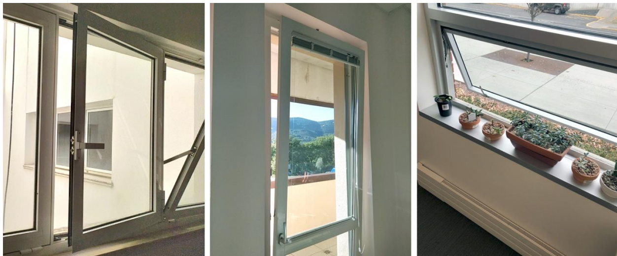
Figure 2: Different examples of operable windows: Single wing window with handle (left); Dual-tilt window in bottom-hung configuration (center); Top-hung window (right).
